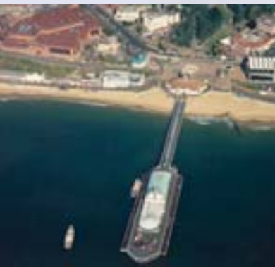
Bournemouth International Centre and Bournemouth Pier
